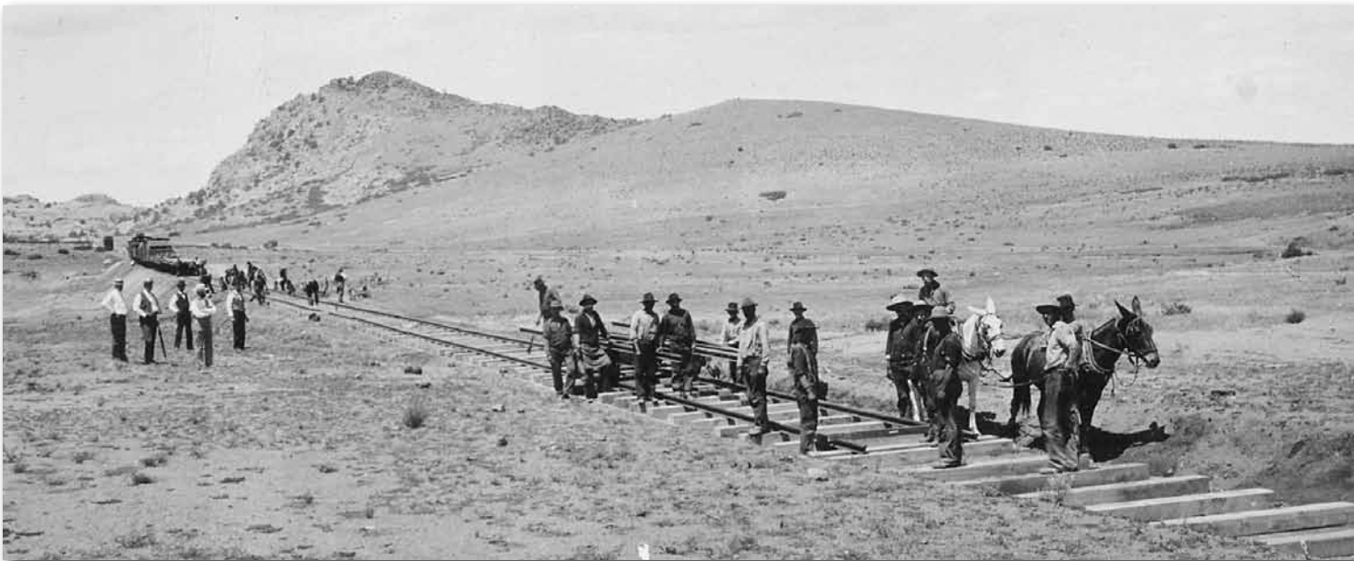
Laying tracks on the extreme front of Prescott and Eastern Railroad in Arizona Territory, ca. 1898.
